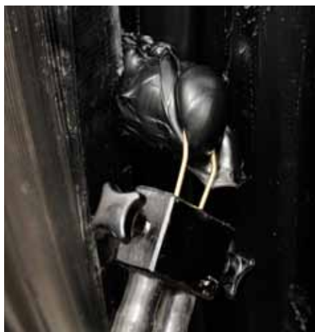
Fig. 4.5.4 Visible sign of welding completion
