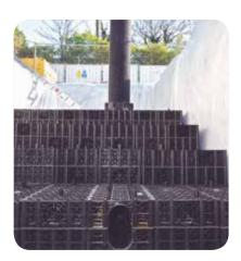
Polypipe's Polystorm Access and Inspect products were used in conjunction with Polystorm-R modular cells to create a 96m<sup>3</sup> structure.
