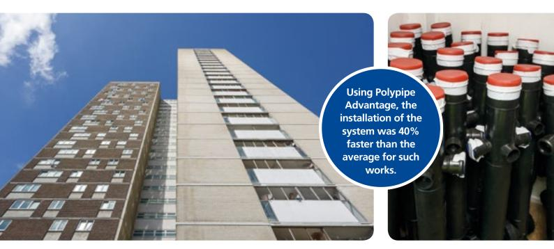
Formerly the tallest building in Southampton, the Millbrook Tower stands at 240 feet. Built over 50 years ago, the building had a cast iron drainage system installed that had started to rust and fail, causing excessive leaking in the 144 flats in the development.
