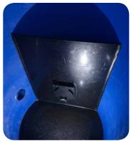
Ridgistorm-XL was supplied in a variety of stiffness classes in order to provide a robust solution to compensate for the varying ground conditions found on-site, including soft clay soils, as well as loading above from vehicles.
