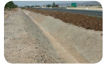
Channel & Stream Protection
