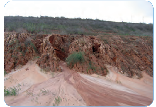
Embankments / Slope Protection
