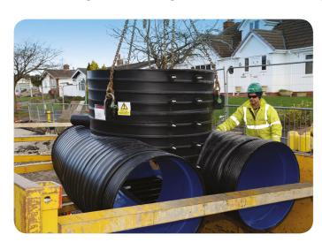
As well as providing Ridgistorm-XL pipes in 900mm diameters, we were able to pre-fabricate structural components to create a number of 1500mm RIDGISTORMAccess Multiple Pipe Manholes, allowing duel carrier pipes to run parallel to one another. The manhole access was positioned centrally to allow for a single point of access into both pipelines.
