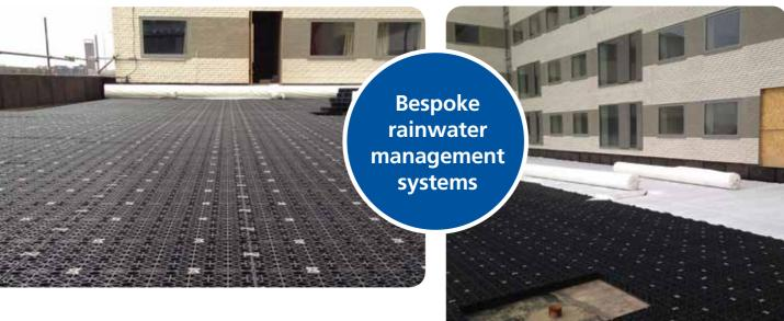
Working alongside main contractor Westfield Construction and M&E contractor Dimension Data Advanced Infrastructure, Polypipe Terrain helped to develop a rainwater attenuation system capable of managing the site's drainage requirements in the event of a '1 in 100' year + 30% storm event.
