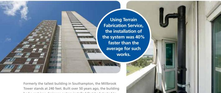
had a cast iron drainage system installed that had started to rust and fail, causing excessive leaking in the 144 flats in the development.
